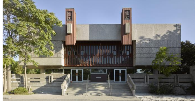
Figure 5. The Old Japanese Canadian Cultural Centre, Toronto, ON. Photo by Moriyama & Teshima Architects.
